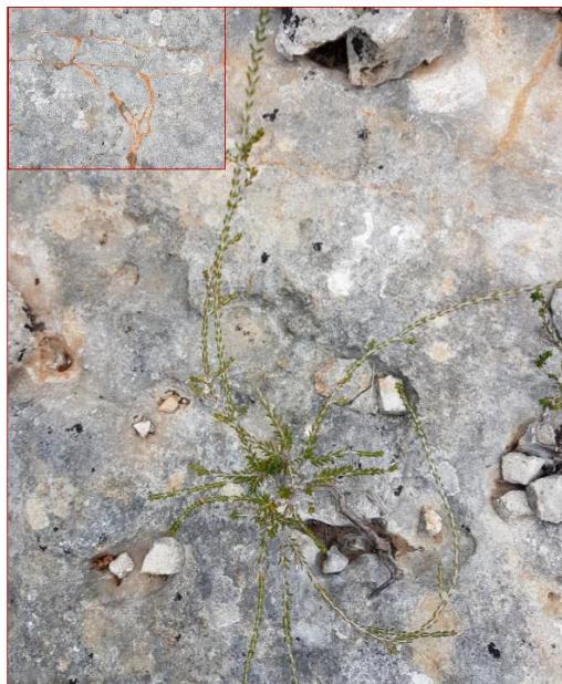
Figure 7: Marine, shallow-water, bioclastic, massive, highly cemented, sandy-carbonates of the Akrotiri Formation with Red-algal fragments. An aromatic, Rosemary evergreen shrub, native to the Mediterranean region is grown along thin joints (cracks) that developed after recent tectonics affected Crete and were secondary filled in with Terra Rosa material (see upper left inlet). Technical University Campus outcrop, Akrotiri, Chania.
